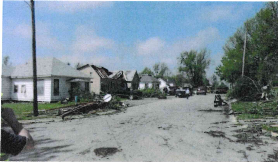
Damage due to twin tornados in Lenox in 2011
